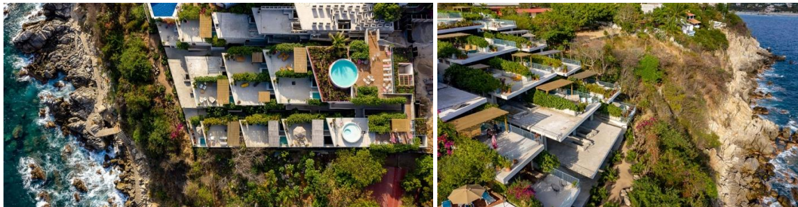
Figure 5. Site plan and elevation of La Escondida Apartments. Photo credit: Onnis Luque, Mauricio Guerrero La Escondida Apartments / Francisco Pardo Arquitecto, (2020).
