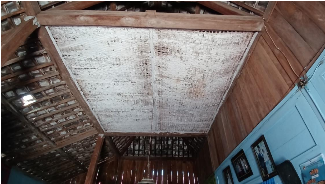
Figure 8. Bamboo ceiling in the Dalem room of the Sinom house. Source : Personal documentation(2024).
