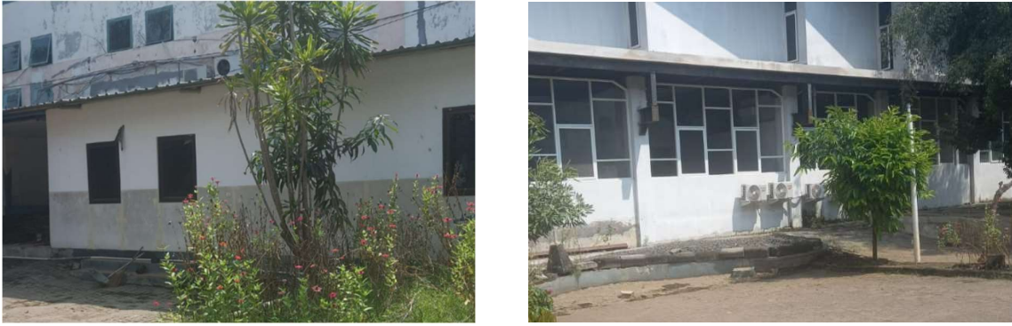
Figure 1. Terang Bangsa Elementary School Existing Condition (Source: Author's Documentation, 2024).
