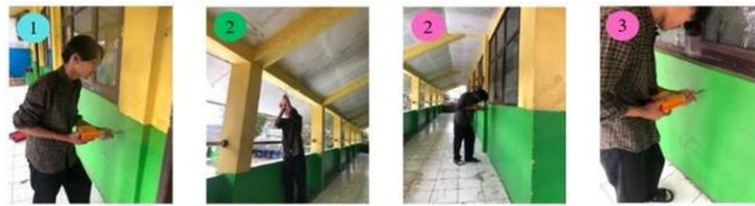
Figure 9. The Hammer Test Process at SDN Barukai (Source: Personal Documentation, 2025).
