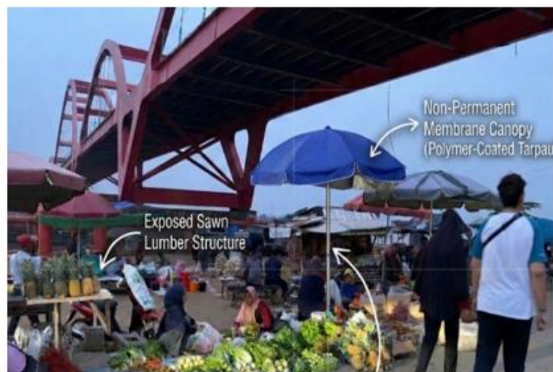
Figure 7. Stall structure and materials used by vendors (Source: Author, 2026)
