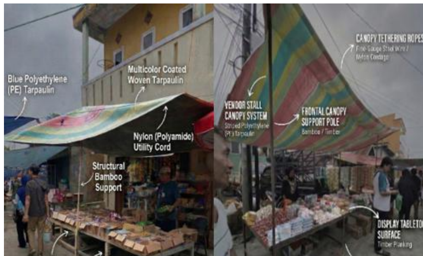
Figure 6. Stall structure and materials used by vendors (Source: Author, 2026).
