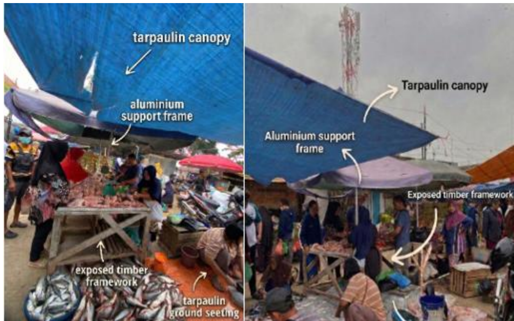
Figure 8. Stall structure and materials used by vendors (Source: Author, 2026).
