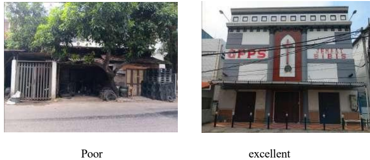
Figure 6. Poor and excellent condition of building facades on Karet Street (Source: Author, 2025).
